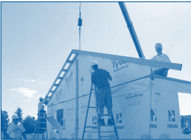
Trusses being set in early August on the Tutt house.
