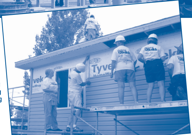
Siding and Roofing Coming Right Along
